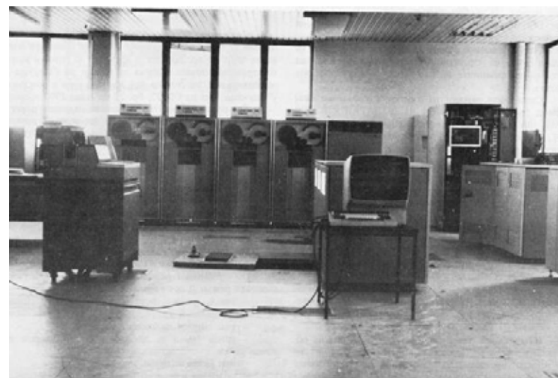
First server room in the Electronic Computer Centre in Belgrade in 1981
